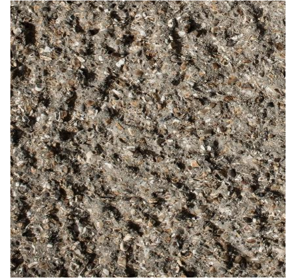
The mechanical treated surface when using colored concrete
