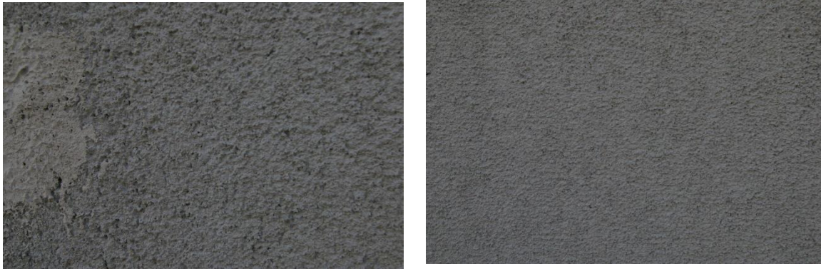
The roller-treated surface when using noncolored concrete
